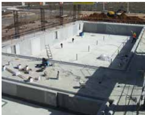
A TOTALLY WATERTIGHT TANK
