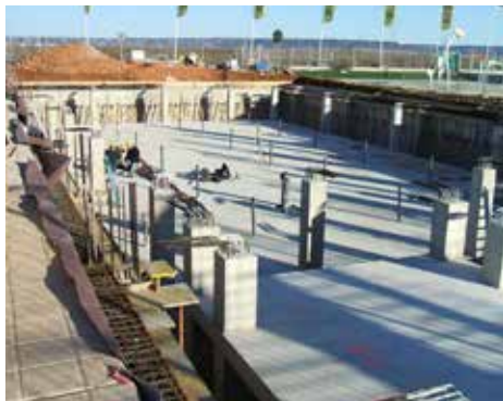
LOAD-BEARING BASE FOR THE PANELS
