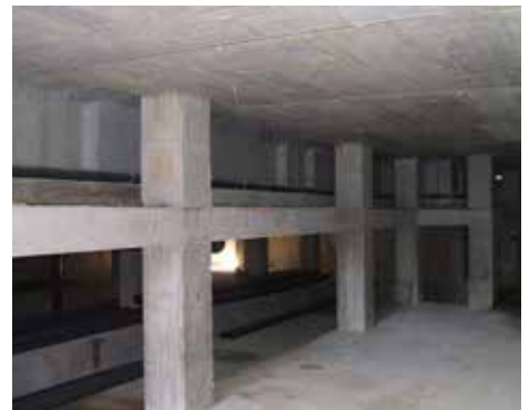
ACCESS TO UNDERCROFT TO THE EXTERNAL FAÇADE OF THE POOL TANK
