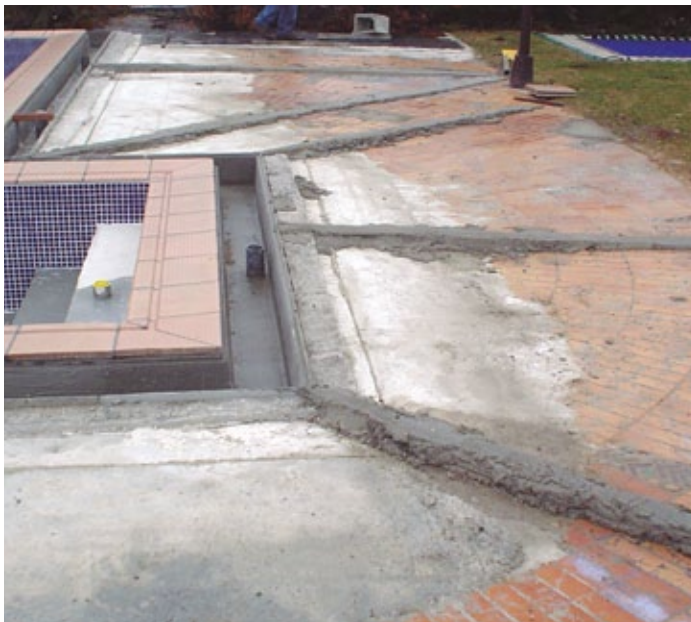
Make load bearing walls to make the slopes
