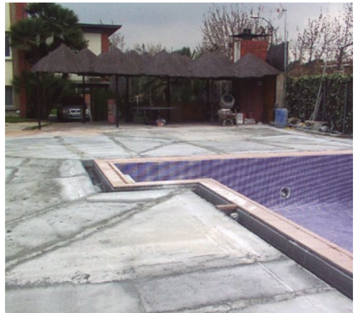
Terrace with the finished slopes before placing the tiles
