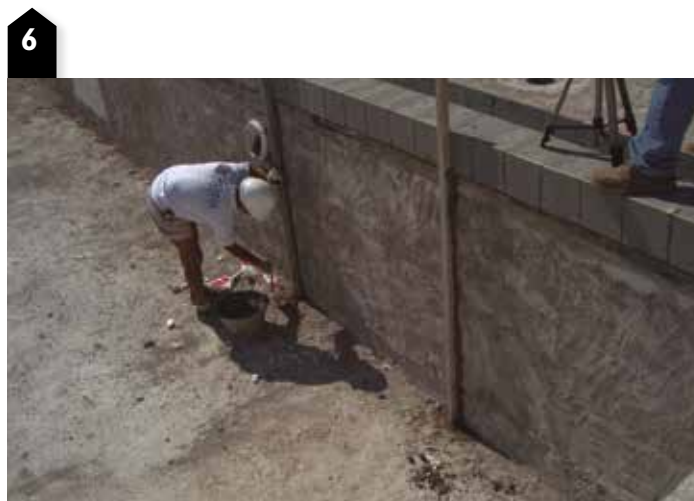
Using the blocks as a guide, the mortar screed from the walls is made with a mortar of uniform quality and quick drying such as FIX-REVOCO .
