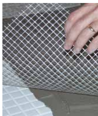
Placement of NET-MORTER-110 mesh
