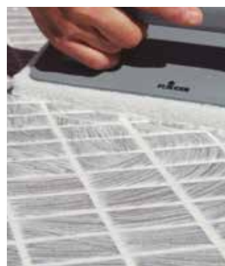
First clean with the trowel and then clean with a soft rag
