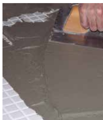
First layer of FIXMAX S2
