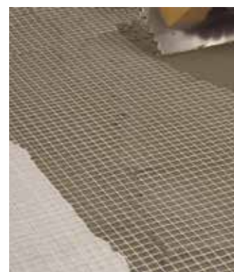
Covering the mesh with FIXMAX S2
