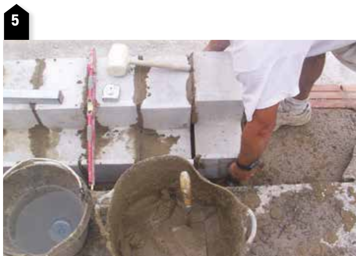
It is also essential to place mortar in the joint between the blocks. Once the blocks have been positioned the back gap is filled with concrete.
