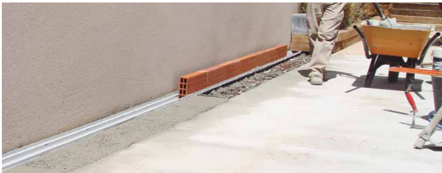
View of the PVC gutter positioned during the mortar-filling phase
