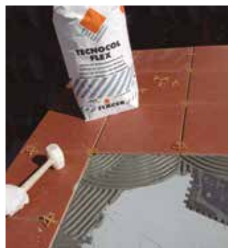
Gluing of the tiles with TECNOCOL FLEX
