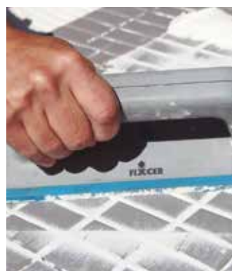
Grout the tile using FIXSET FLEX
