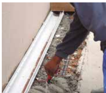
Placing the mortar around the channel
