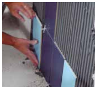
Set the slabs with TECNOCOL FLEX
