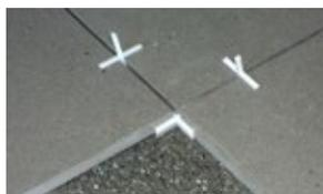
**05** We use non-recoverable 2 mm cross-shaped spacers. The spacers serve to homogenize both the width of the assembly and as fastening for the tiles. They remain permanently in place.
